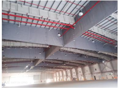
NAFFCO Static Smoke Curtains are a reliable solution for offering smoke protection in commercial and industrial buildings. Draft curtains, which are secured to structural steel, ensure that smoke and hot gases emitted during fire remain buoyant within the smoke zone, in accordance with smoke management strategies.
